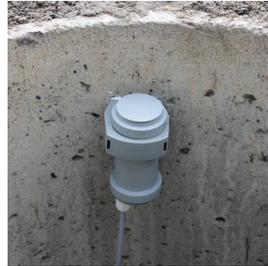
Placing the sensor in the tank is suitably in the sleeve on the tank. The sensor has a 1" connection. Height tank is adjusted by sliding the sensor to the desired position and fixed by tighten the adjustment screw in 1" terminal. Depending on the type of tank/neck tank sensor may have to be mounted in other ways. For instructions, contact the tank manufacturer. See examples below.
